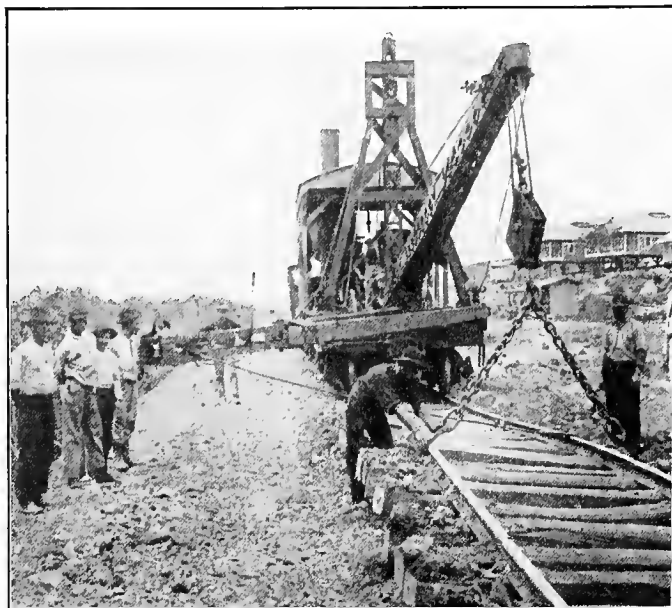
THE TRACK SHIFTER IN ACTION
